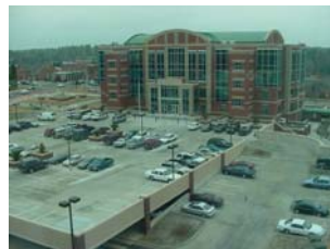
Lexington County Administrative Complex
